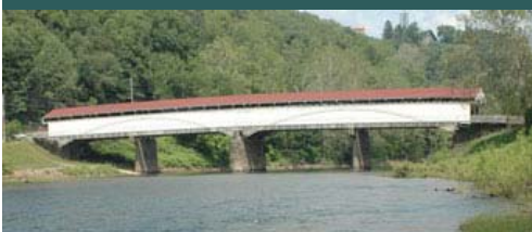
Philippi WV—Covered Bridge
